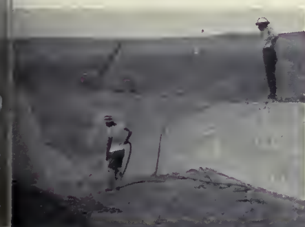
OUTH DAM'S CONCRETE CORE (below) with "Pot" O'Donnell supervising men to the who is cleaning up the bedrock. At center, below, the old highway through the and Coulee as the water gradually rose in the ice-age channel of the Columbia r. A new highway skirts the east wall of the Coulee. At right, O'Donnell is erfed by the giant outlet channels which release water from South Dam into the h Canal of the project. Photos below by H. W. Fuller, photo at right by F. B. eroy. Both are Region 1 photographers.
